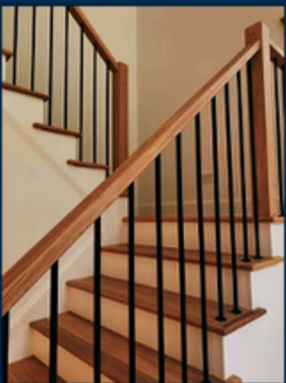
STAIRCASE DESIGN OAK HANDRAIL/NEWEL POST/TREADS – STAINED TO MATCH FLOOR BLACK IRON BALUSTERS – ROUND OR SQUARE RISERS/STRINGERS – PAINTED TO MATCH TRIM COLOUR
